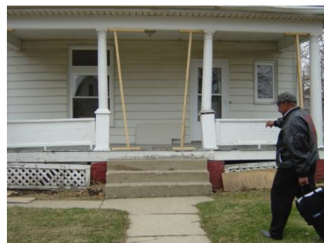
Project Porch Restoration
